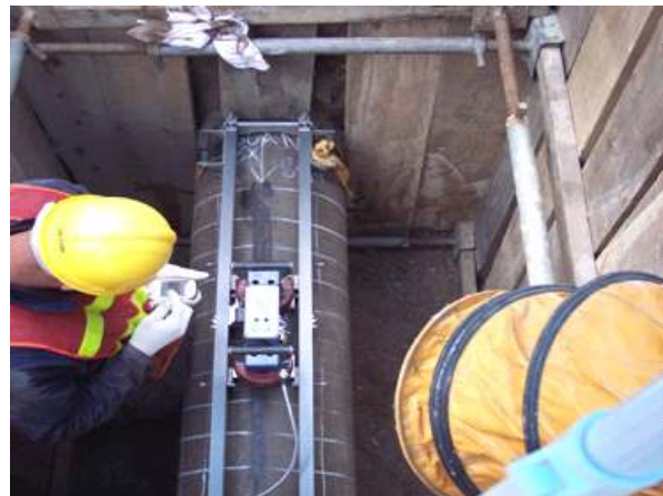
LARGE DIAMETER PIPELINE INSPECTION
